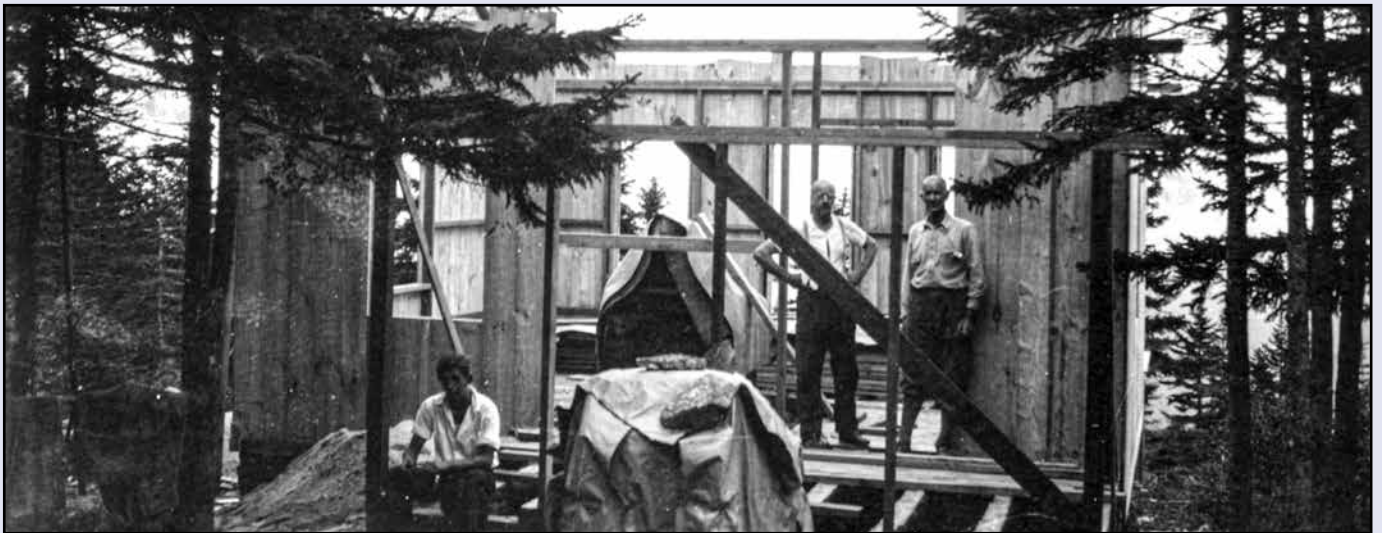
September 11, 1931: Things are beginning to take shape. The floor is in and the walls are going up. AMC Archives.
